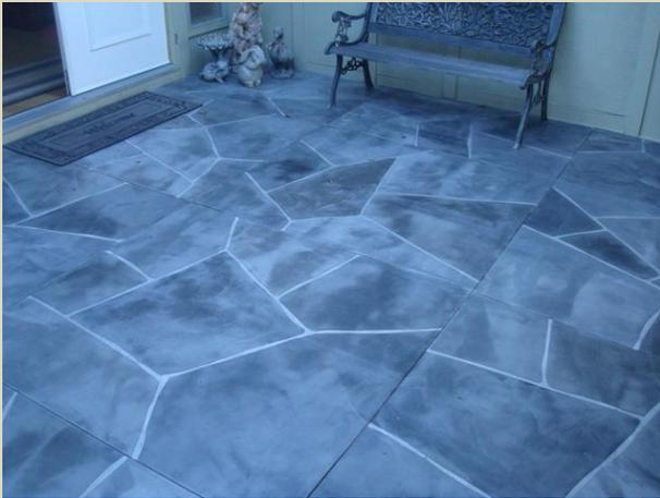
**Sealer** – Stained concrete must be sealed to prevent accidental staining and contamination of the surface. The sealer will also extend the performance of the stain by protecting the surface from fast wearing. The frequency depending on the sealer selection, maintenance applications are normally necessary to maintain the aesthetics to top levels of performance.
