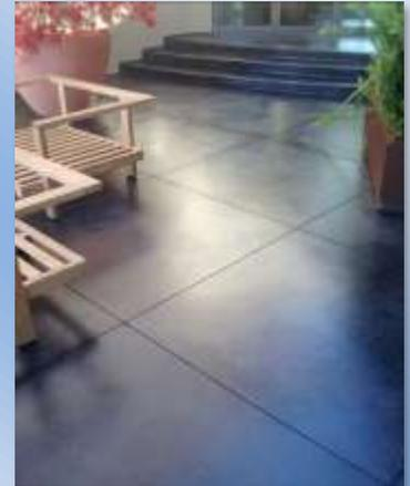
**Polished coatings and Self-leveling coatings** – Whenever the structural conditions of the existing floor slab are not suitable for a direct polishing, a new layer of engineered cement can be applied to the surface and then ground and diamond polished. This process is a multi-phase installation that allows for total customization (glass chips, integral colors, metallic inlays...) and creates an incredibly attractive and durable floor.
