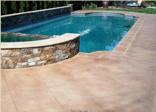
**Color selection** — Most manufactures supply a color chart to select the desired color. The color chart should be used to select the “pigment”, not as a representation of the final look and tone. Many factors such as color of the existing concrete, porosity, chemical composition and density of the slab, will contribute to the final appearance. We highly recommend whenever possible to prepare mockups for proper preview.
